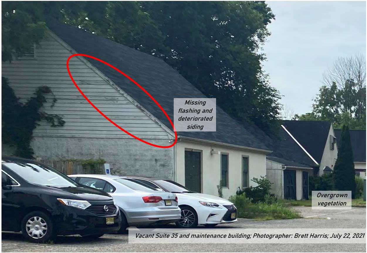
Missing flashing and deteriorated siding
