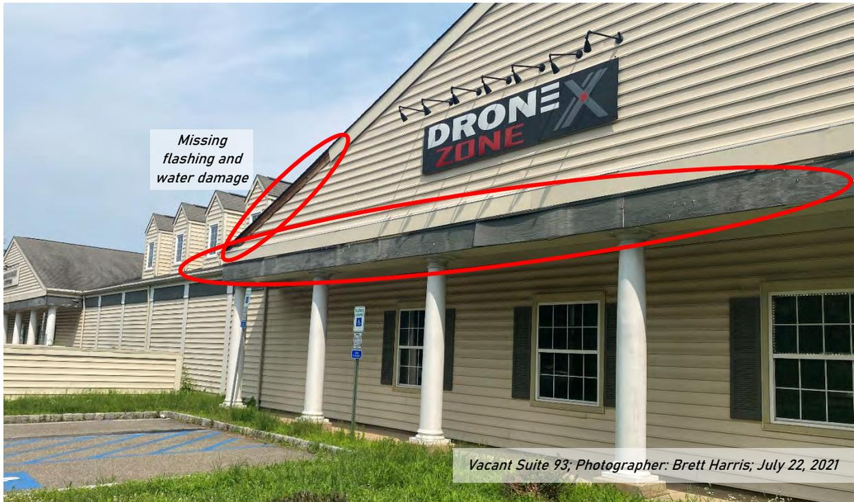
Missing flashing and water damage
