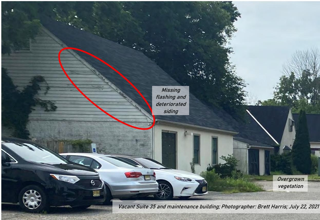
Missing flashing and deteriorated siding
