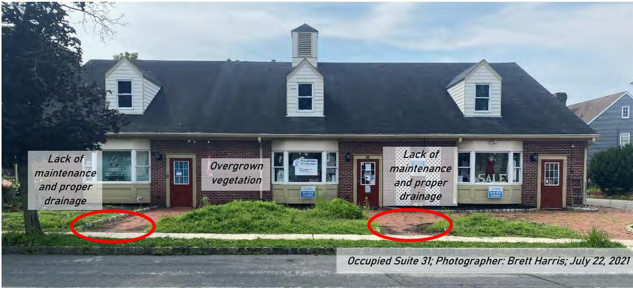
*Lack of maintenance and proper drainage*
