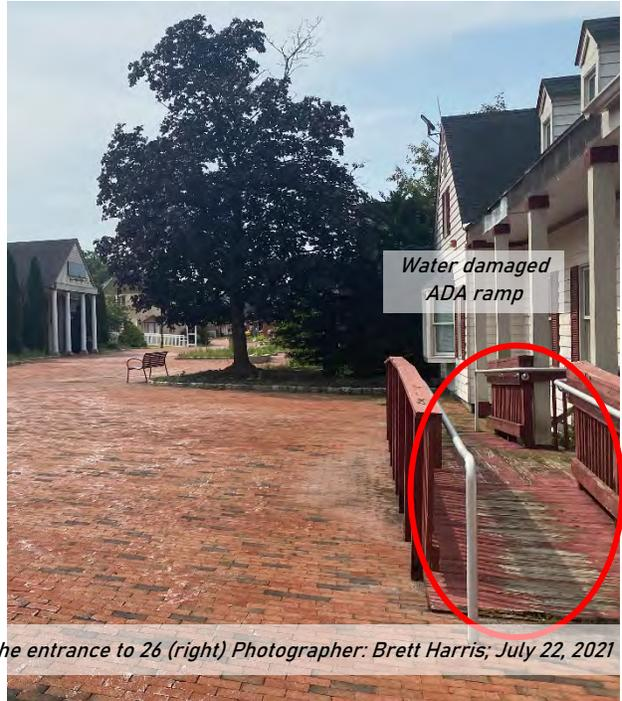
*Water damaged ADA ramp*
