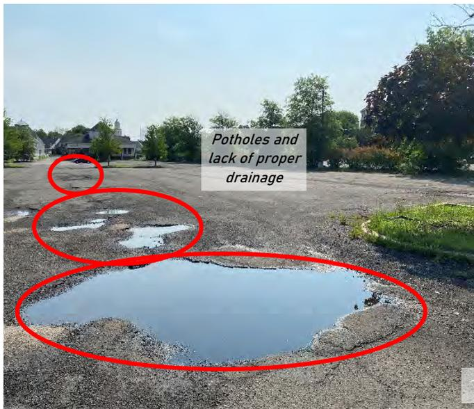
*Potholes and lack of proper drainage*
