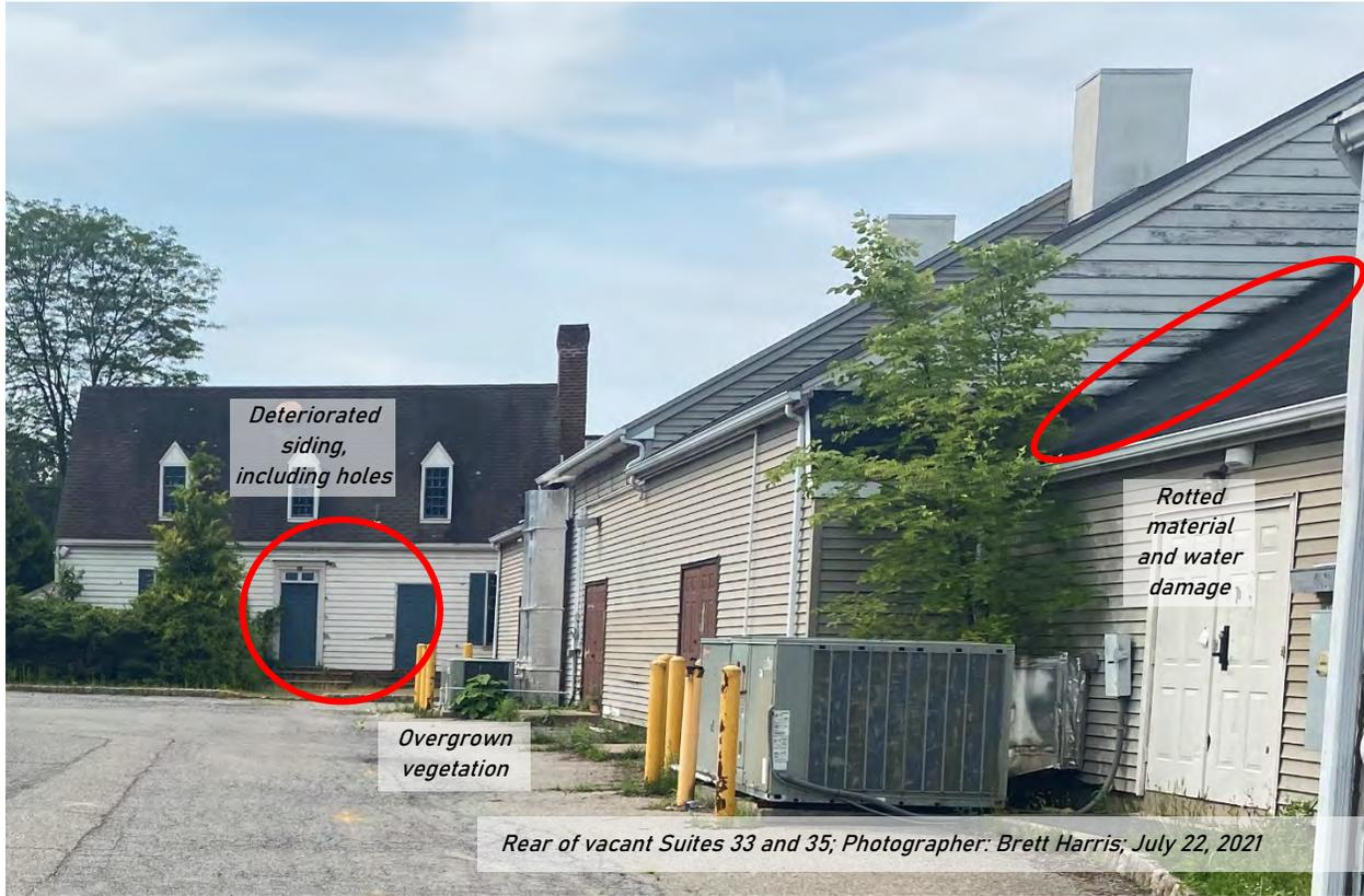
*Deteriorated siding, including holes*
