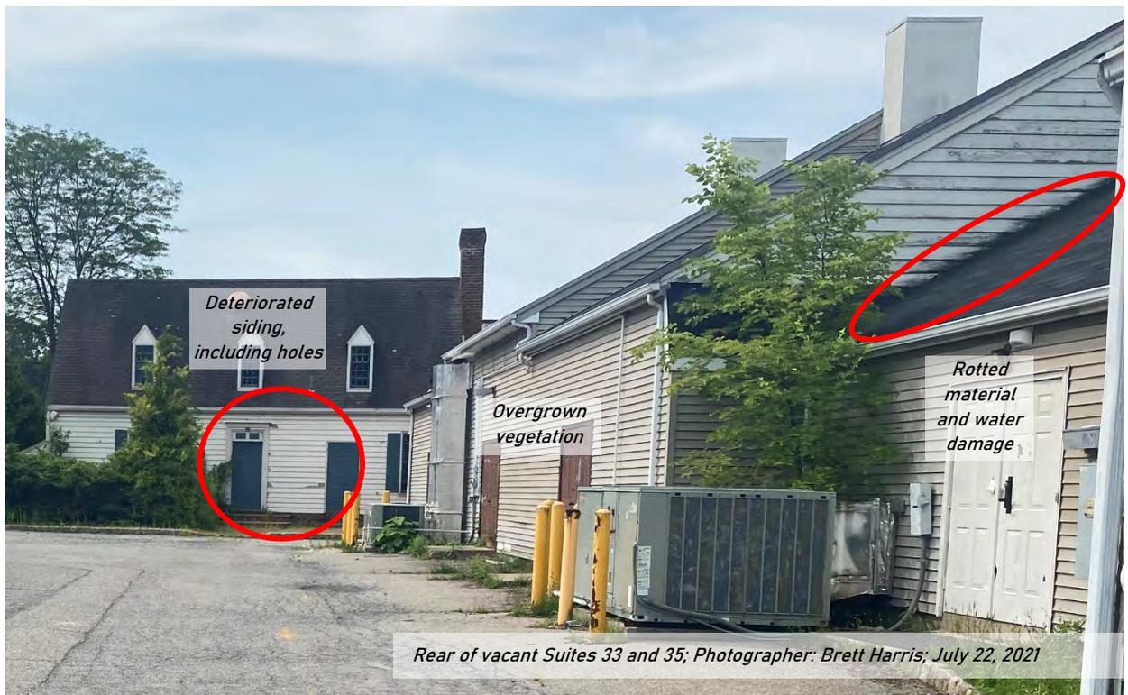
Deteriorated siding, including holes
