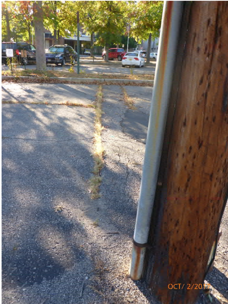
Plate 3-5: Evidence of belowground electrical cable traversing southern end of parking lot.
