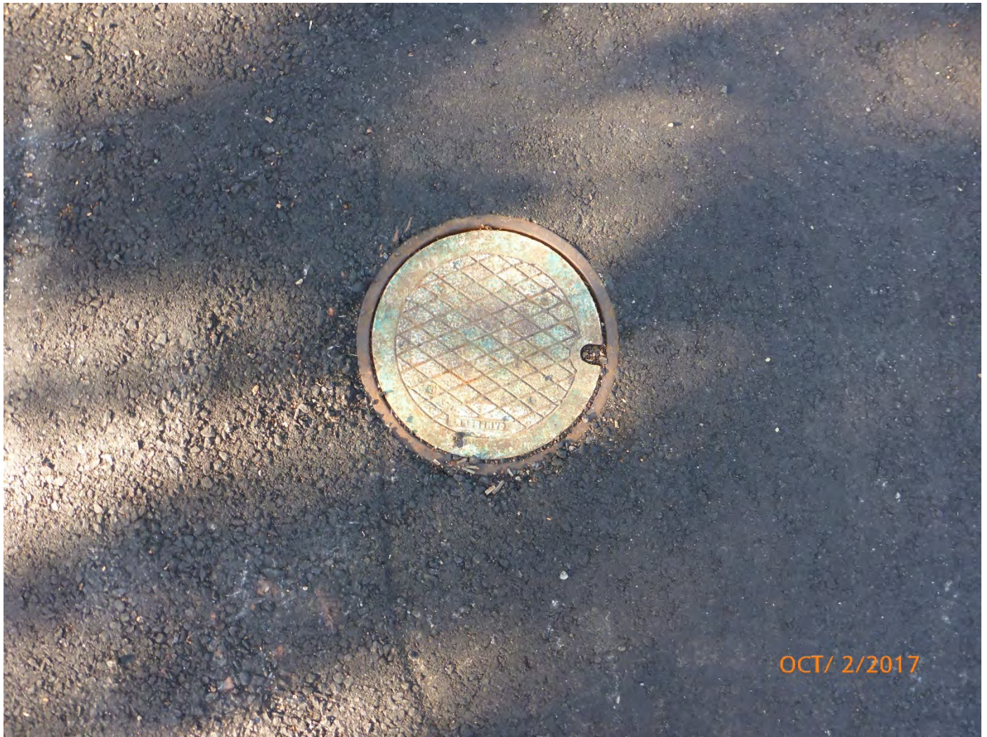
Plate 3-12: Gas access cover in parking lot. The location of the attached pipeline is not evident from surface indications.
