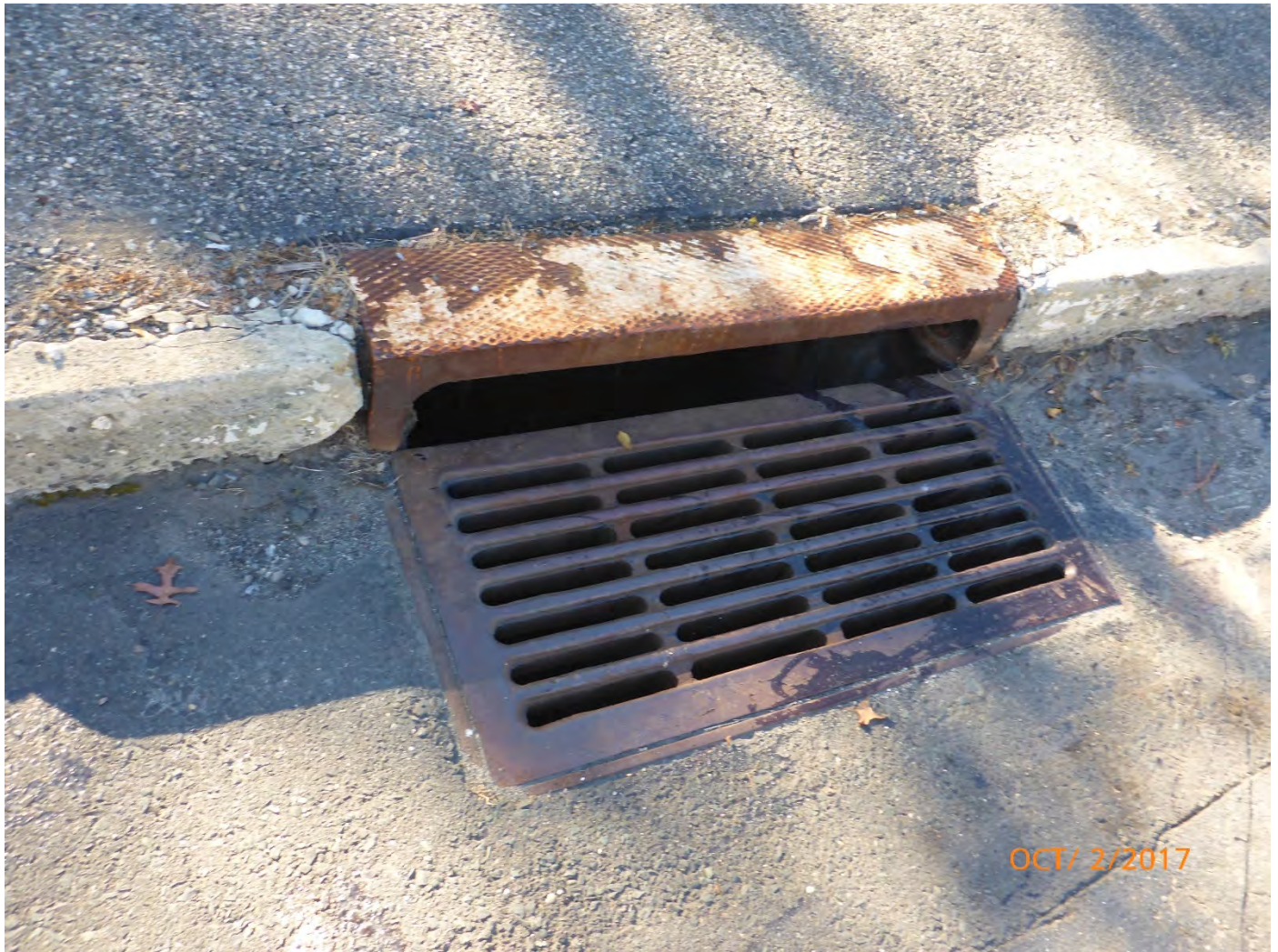
Plate 3-8: Storm sewers are present along the west side of each parking lot island.
