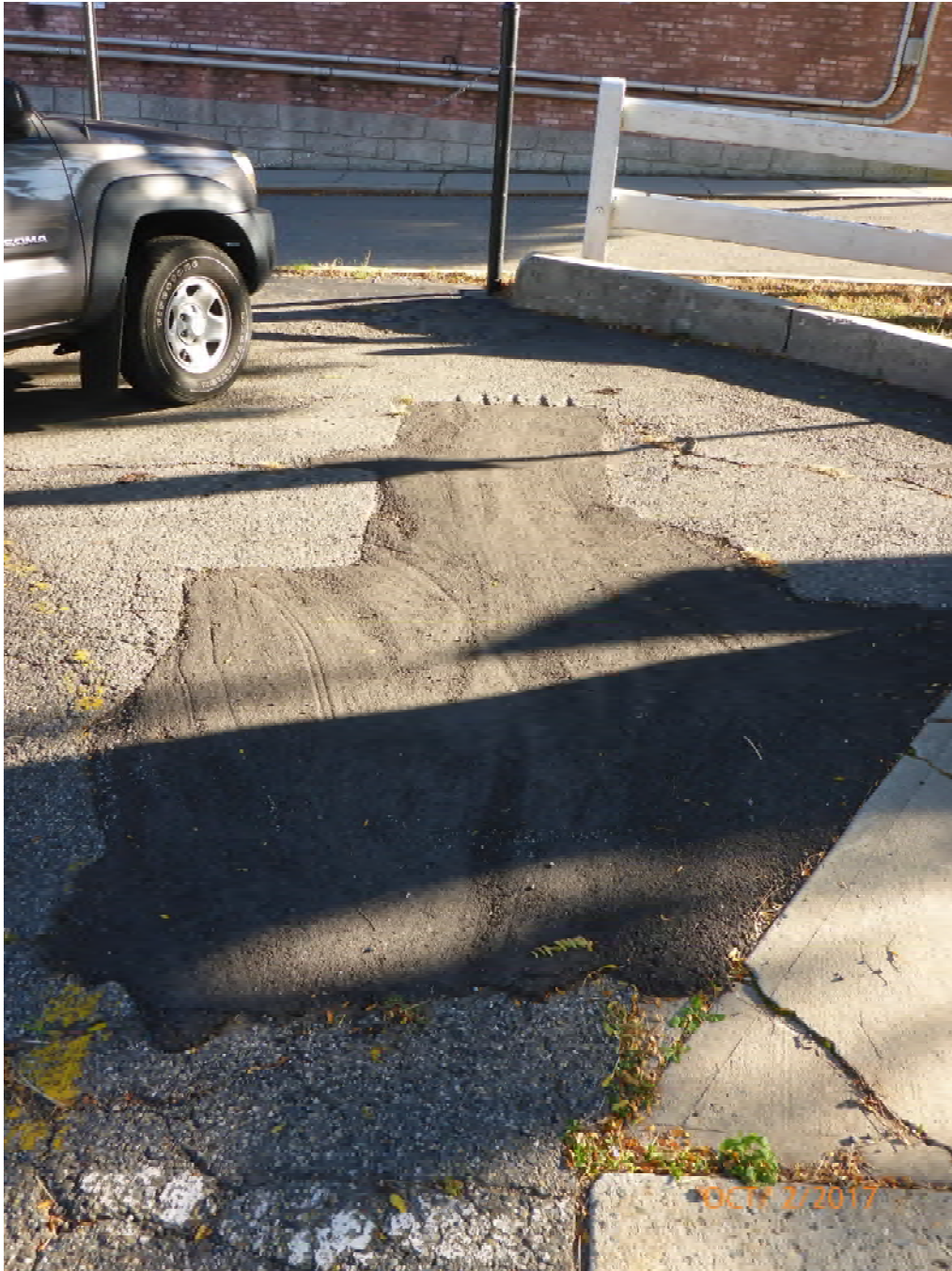
Plate 3-7: Example of existing excavation and parking lot repair.
