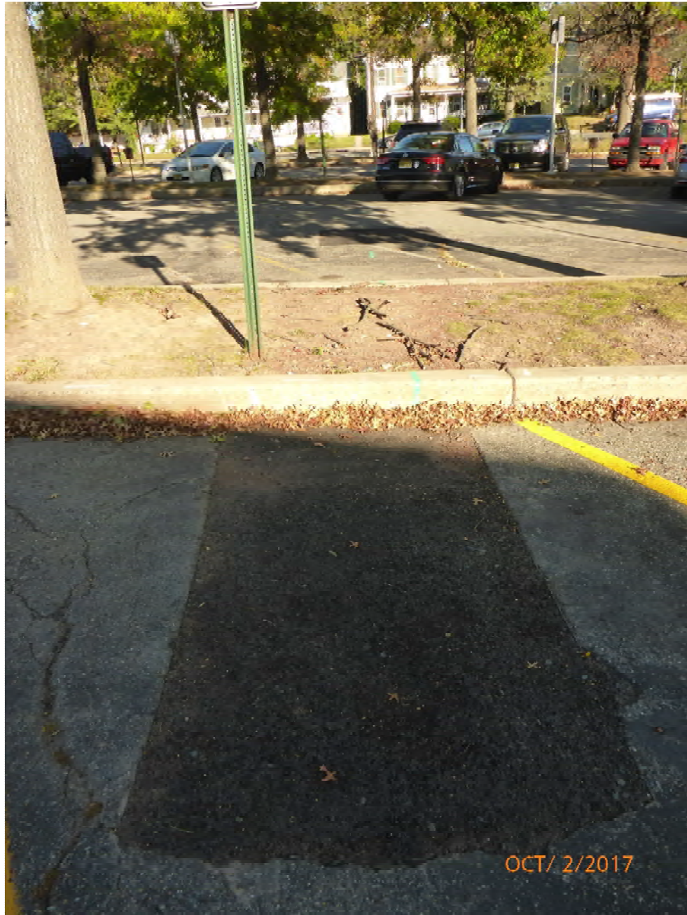
Plate 3-6: Evidence of unknown utility emplacement or other excavation and repair.
