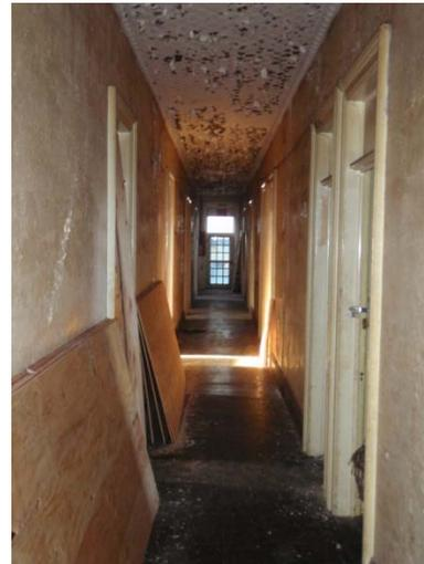
The fourth floor is attic space that has never been occupied. The roof structure is in good condition, although there is some evidence of minor water damage. The space is quite tall and open and could be readily renovated for other uses.
