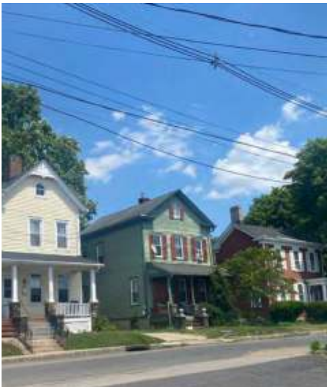
Single family homes on Main St
