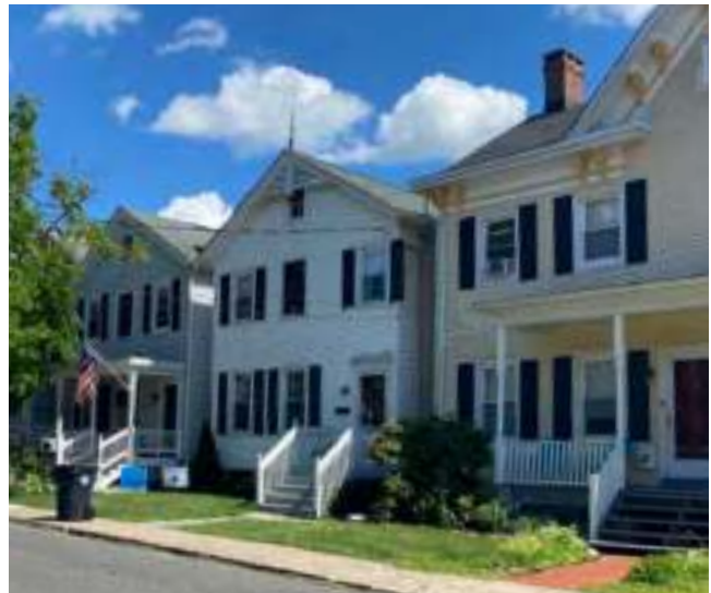
Single & two-family homes along Court St
