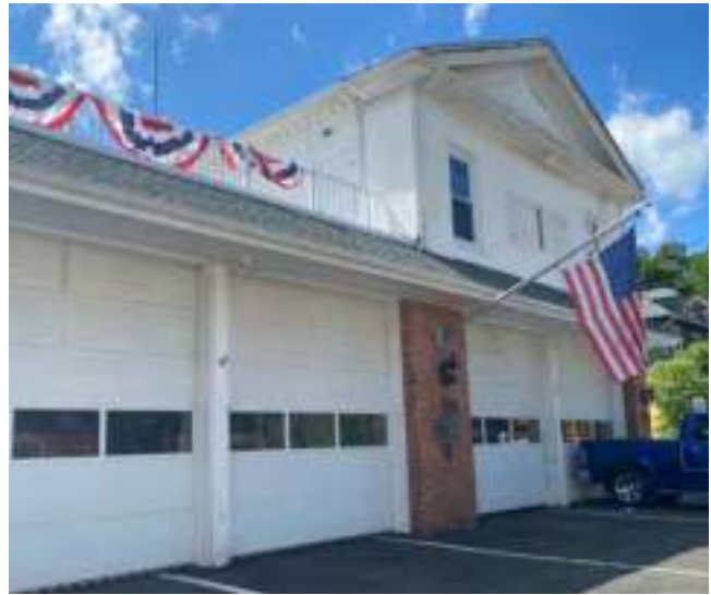
Flemington Borough Municipal Building
