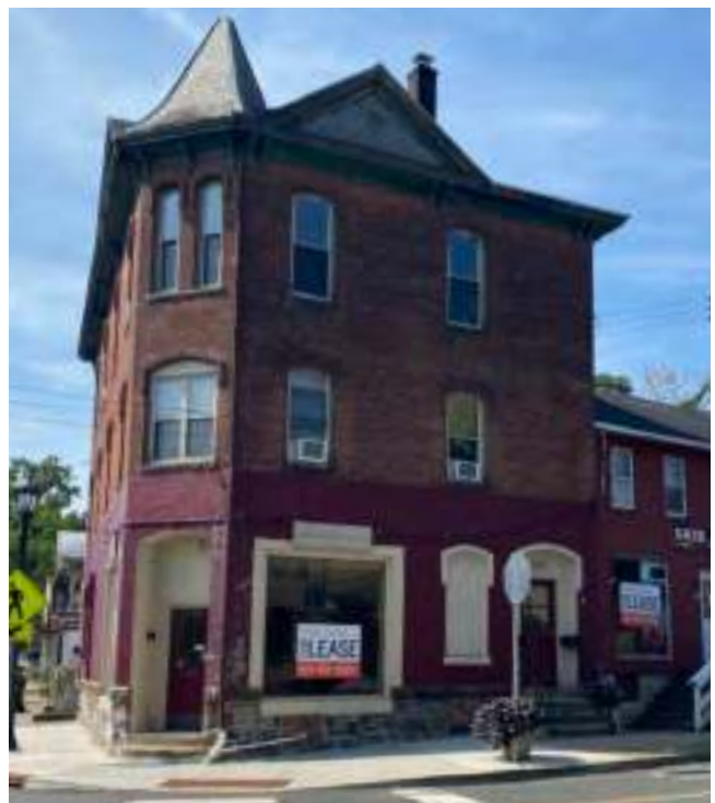
Vacant historic building on Main St
