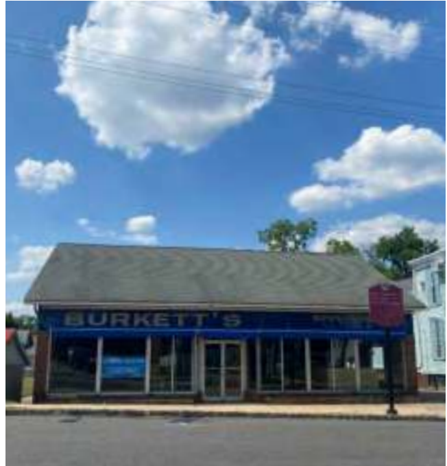
Vacant commercial use in DBII District
