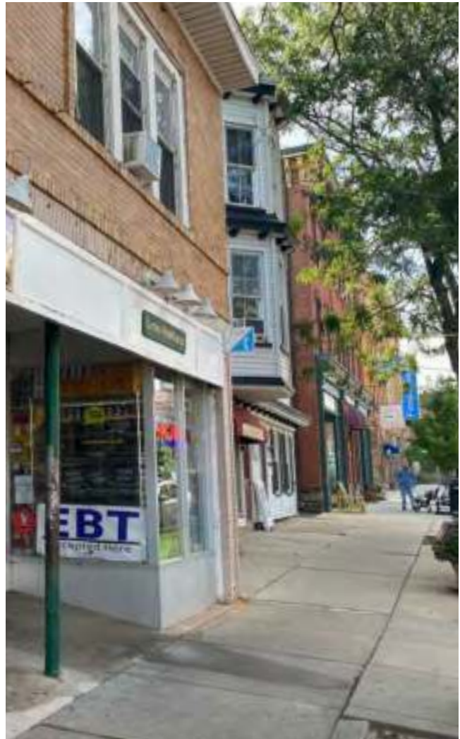
Main St building facades
