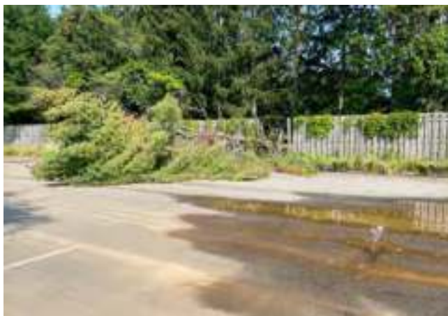
Fallen tree & water in Liberty Village parking lot
