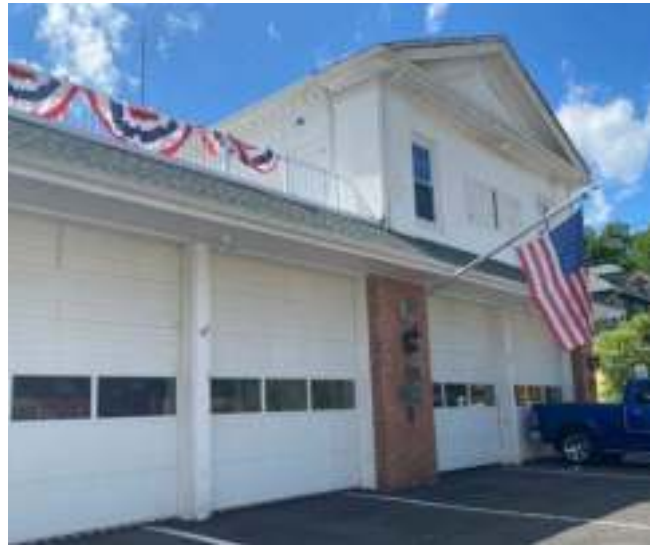
Flemington Borough Municipal Building
