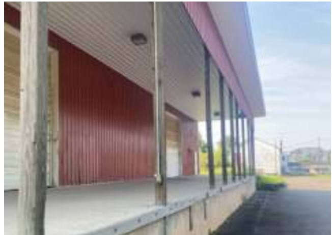
Building in Global Agway RD Area
