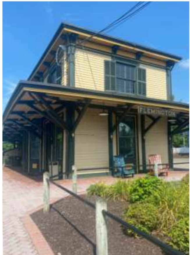
Historic train station on Main St.
