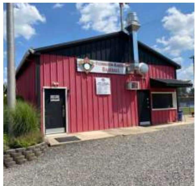
Memorial Field concession building
