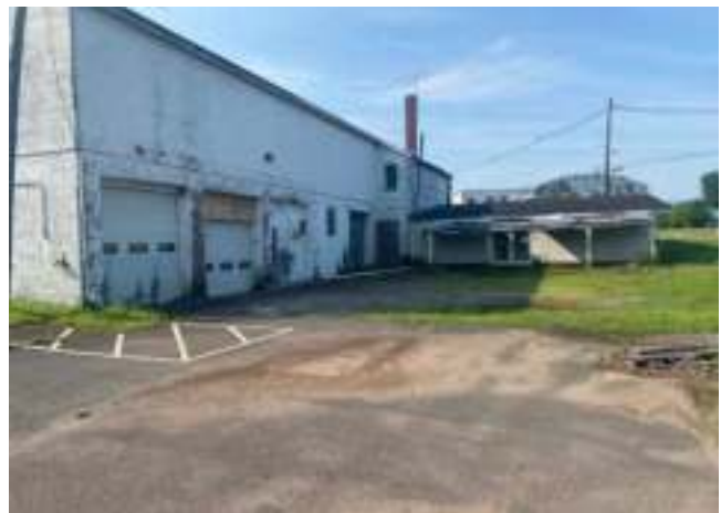
Building in Global Agway RD Area
