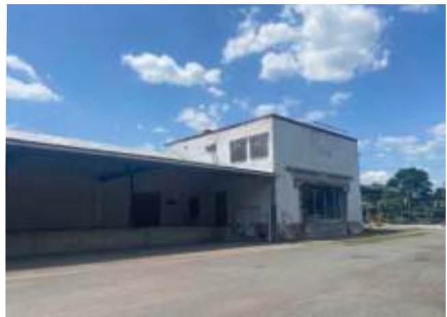
Building in Global Agway RD Area
