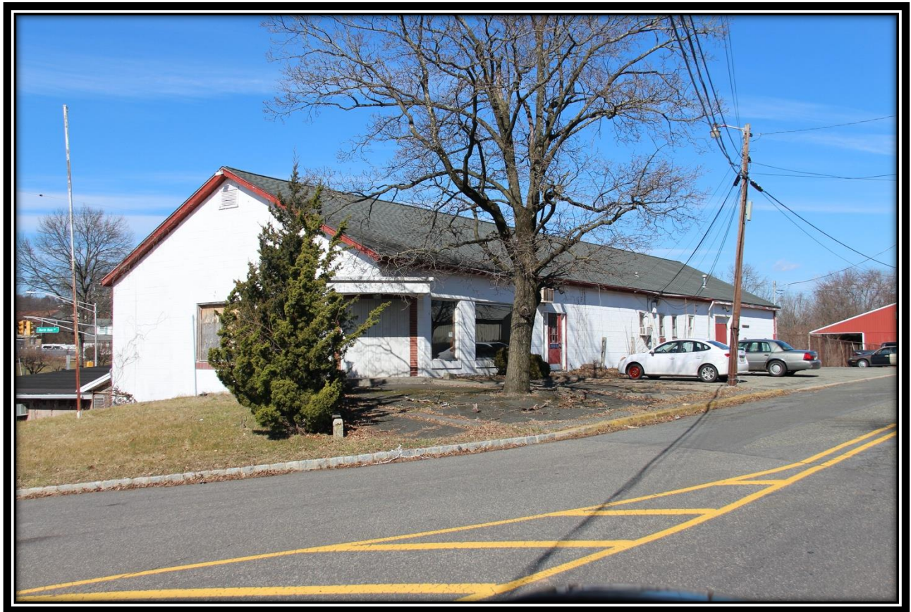
Global Agway Retail Building (view from Hopewell Avenue)
