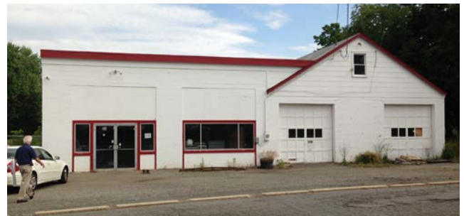
Global Agway (Block 5, Lots 1 and 2) former retail building; view from Hopewell Avenue
