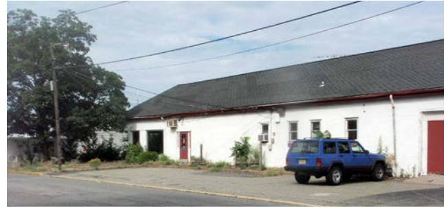
Global Agway (Block 5, Lots 1 and 2) former retail building; view from Hopewell Avenue
