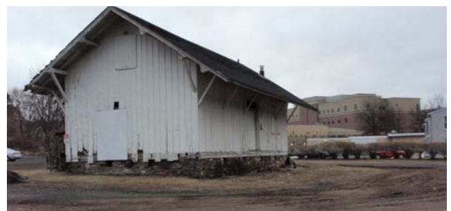
Freight Train Depot (Block 14, Lot 1)
