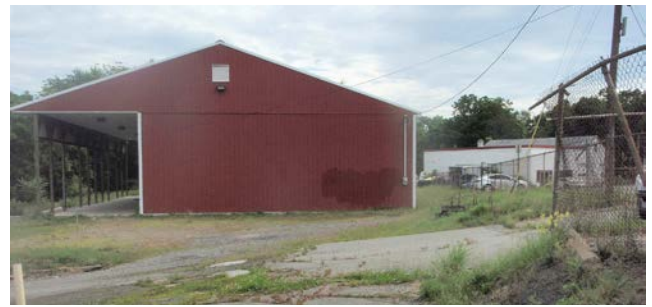
Global Agway (Block 5, Lots 1 and 2) storage building; view from site interior
